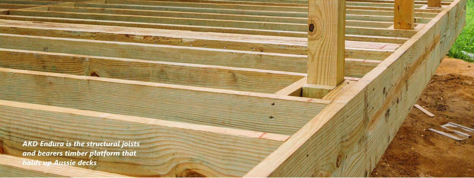
*AKD Endura is the structural joists and bearers timber platform that holds up Aussie decks*
