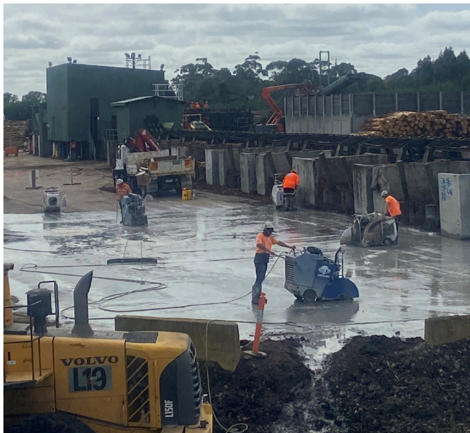
Concrete repair works in front of the Log Deck.
