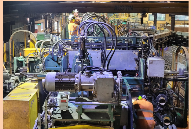
Colac Maintenance team working on the HSS on Good Friday
