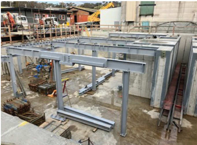
Steel Work for Mezzanine Floor.
