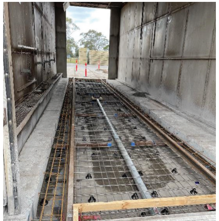
Replacement of kiln railway tracks and drainage system upgrade.
