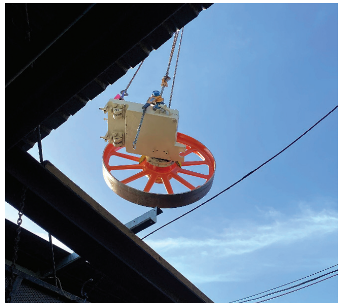
Crane lifting and placing the Top Band Wheel Structure back into place.
